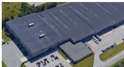
Barrie, ON (CAN) - High Performance Doors
